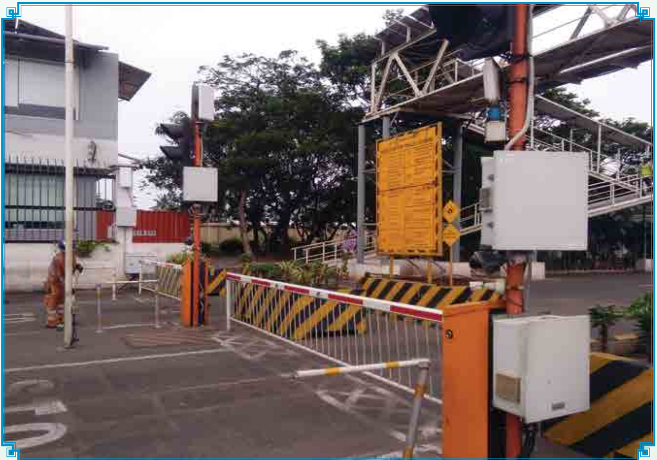
RFID READERS INSTALLED AT TOLL PLAZAS UNDER LOGISTICS DATA SERVICE PROJECT
